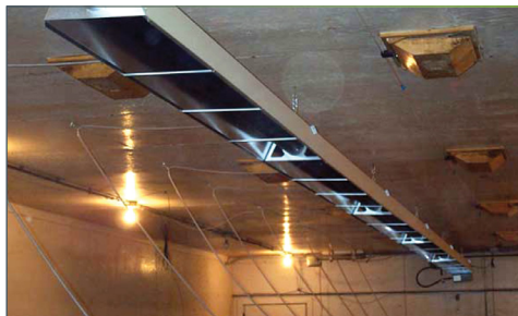
Figure 4. Typical infrared heater Source: Prairie Swine Centre
