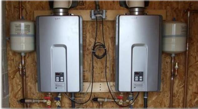
Figure 3: Tankless water heaters usually have smaller natural gas demands
