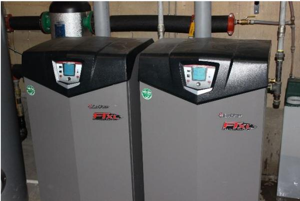
The boiler upgrade consisted of two old 400,000btu Super-Hot boilers (AFUE of 75%-80%) being replaced by two high efficiency 400,000btu condensing and modulating Lochinvar FTXL boilers with AFUE ratings of 95%. AFUE ratings represent how efficiently the heat from the burning natural gas is transferred into the boiler water. The Lochinvar boilers also have a 10:1 turn down ratio, allowing them to modulate the burner temperatures proportional to the barn's needed heat.
