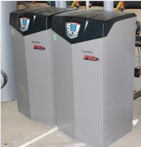
Figure 2: Two High Efficiency Lochinvar FTXL 400,000btu (800,000btu combined) Annual Fuel Utilization Efficiency (AFUE) 95%
